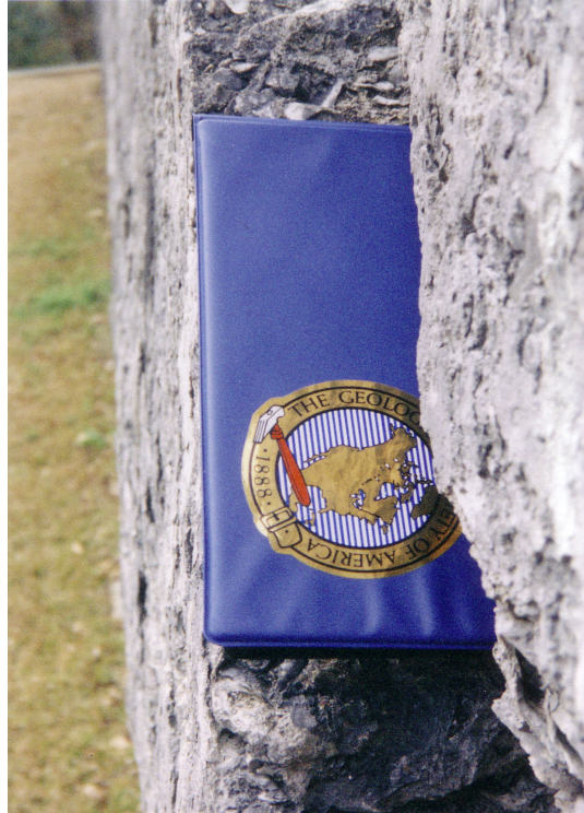
Figure 4b: A left-lateral displacement of 10 cm of the southern wall of Fort Dorchester (Location B in Figure 3, inset).
