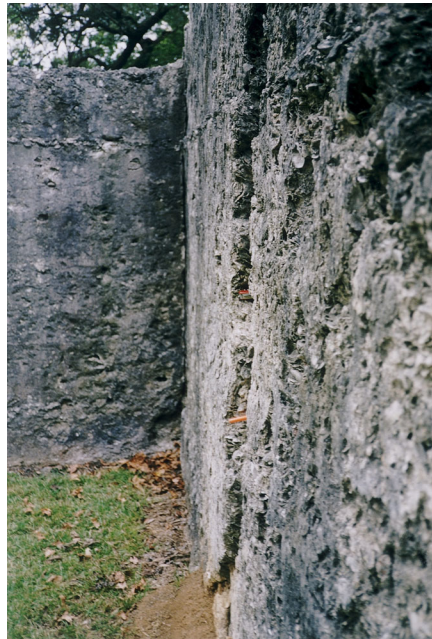
Figure 4a: Left lateral displacement of 7 cm of the northern wall of Fort Dorchester (location A in Figure 3, inset).
